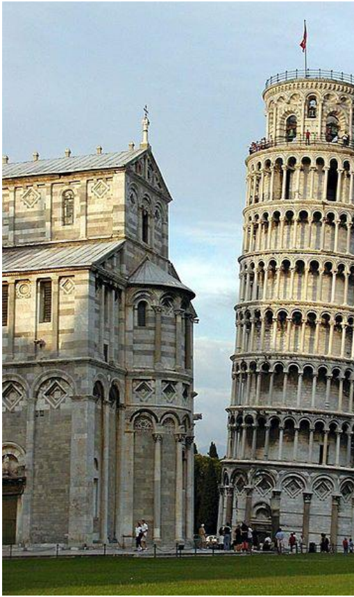
Leaning Tower of Pisa
